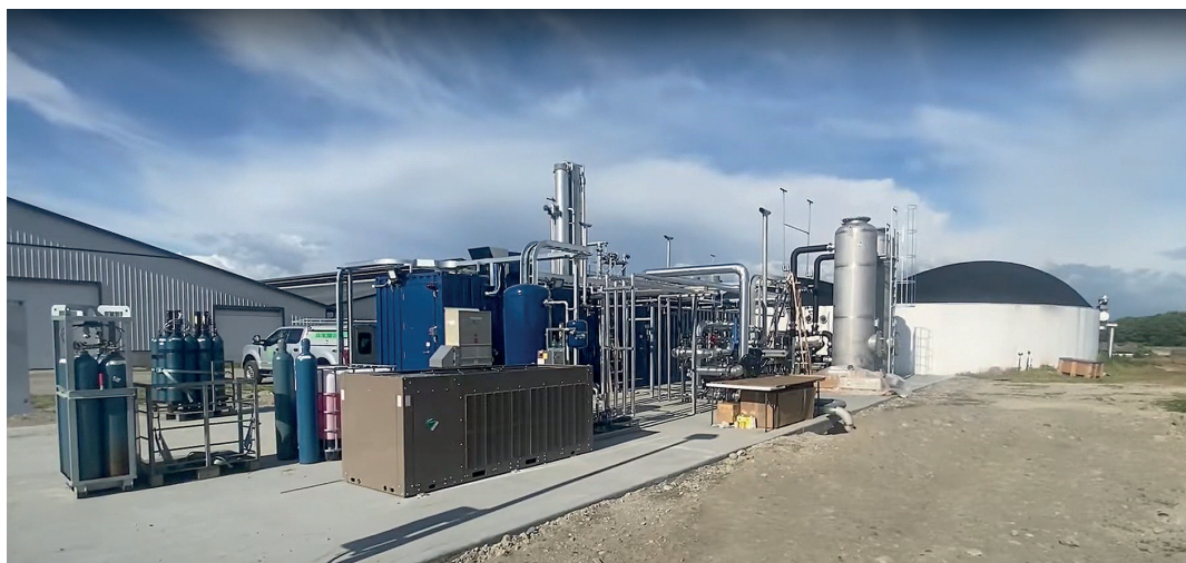
A mid-size dairy farm in British Columbia replaces a water wash system with DMT's Carborex® MS, a membrane separation system, to extract CO 2 from the methane (CH 4 ) stream
