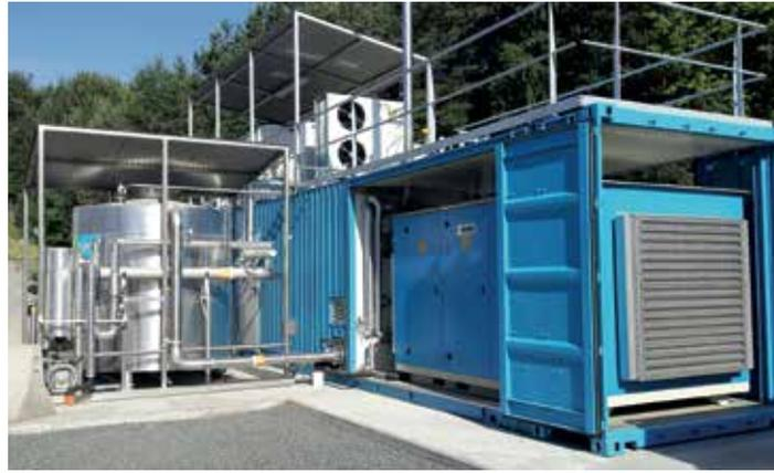
The HRA biogas facility in Jevnaker, Norway uses DMT's Carborex® MS, a membrane separation system to extract CO<sub>2</sub> from the CH<sub>4</sub> stream and upgrades 250 SCFM of biogas into bio-CNG
