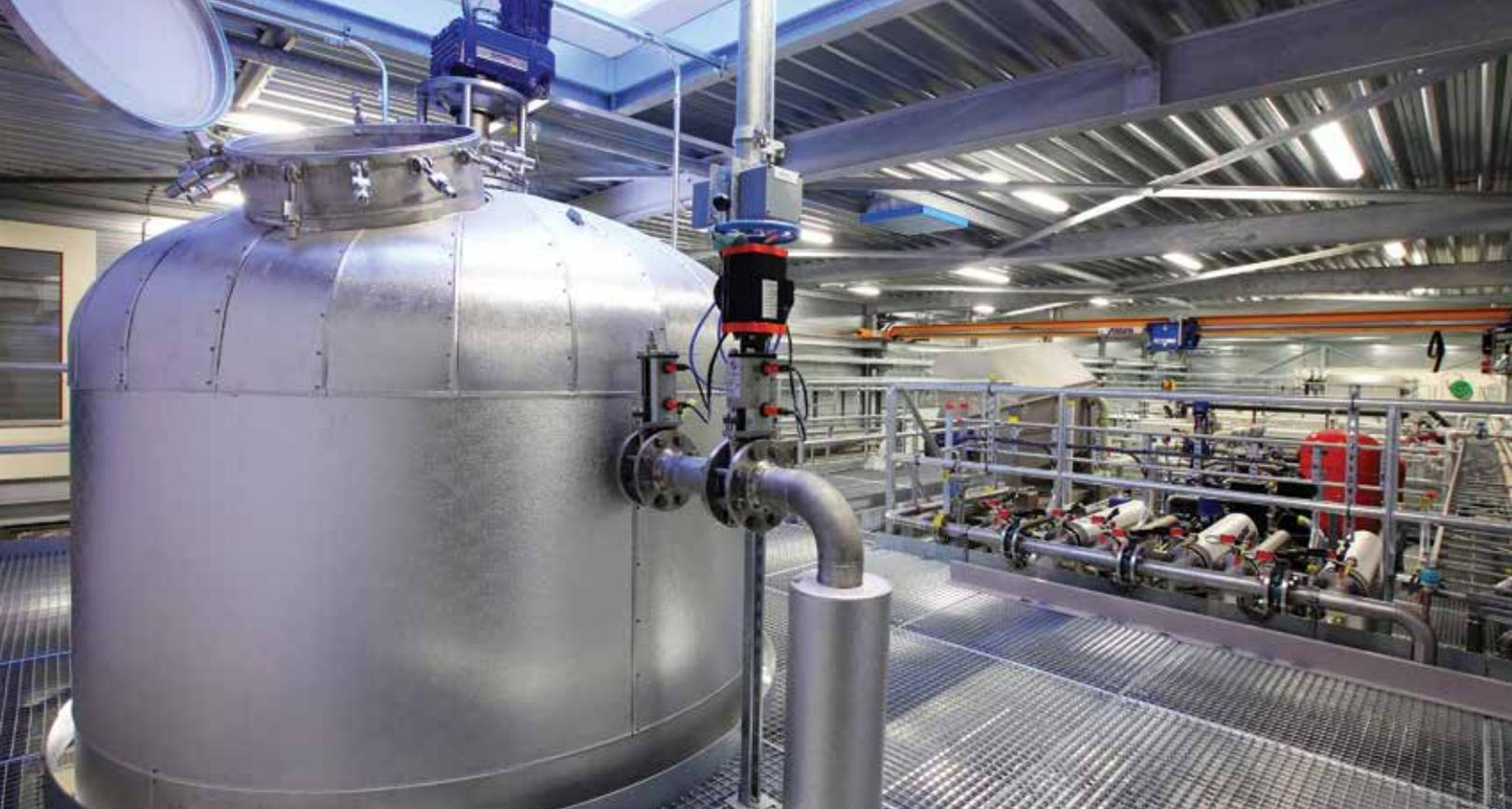
**BIOSOLID BOOST:** Pictured at a wastewater treatment plant, the Turbotec THP reactor couples a mixing and separation technology with efficient heat recovery.
